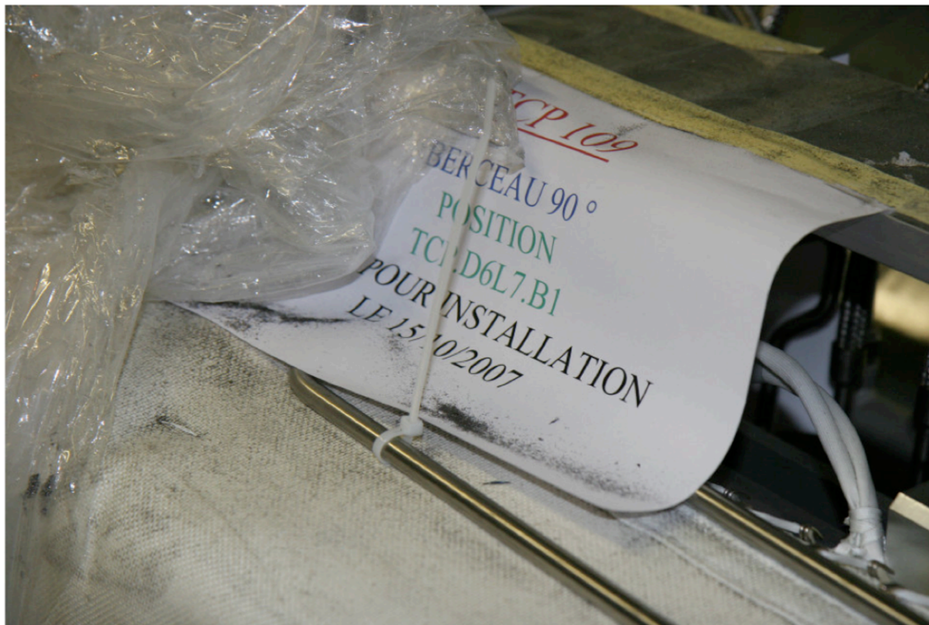
Heavy debris from cutting and welding found on the collimator, its mechanical system and on sensors.
